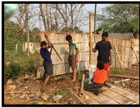
Bamboo boundary wall repair
